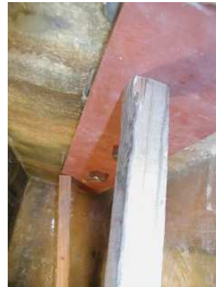
ARG installation surface (bottom view)
