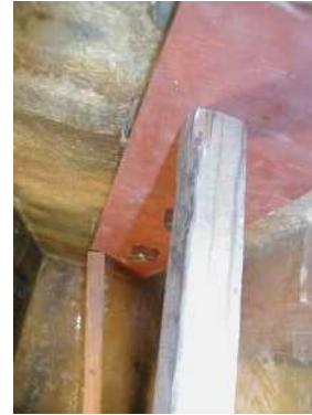
ARG installation surface (bottom view)
