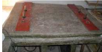
ARG installation surface
