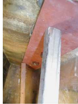
ARG installation surface (bottom view)
