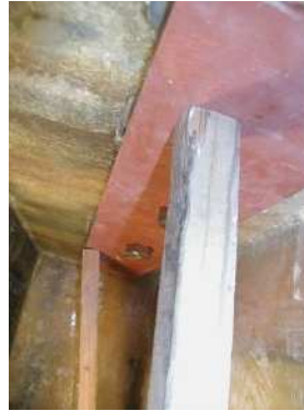
ARG installation surface (bottom view)
