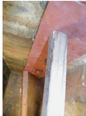
ARG installation surface (bottom view)
